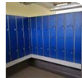
Bricked plinth with protruding bench
